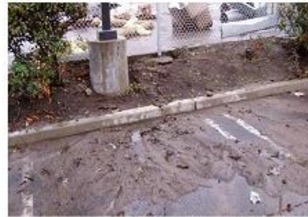
d. Run-on from Parcel 3 to Parcel 2 Causes Erosion of Greenbelt
