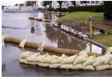
c. Flooding at Parcel 3. Sump Pump Is Required to Remove Ponded Runoff
