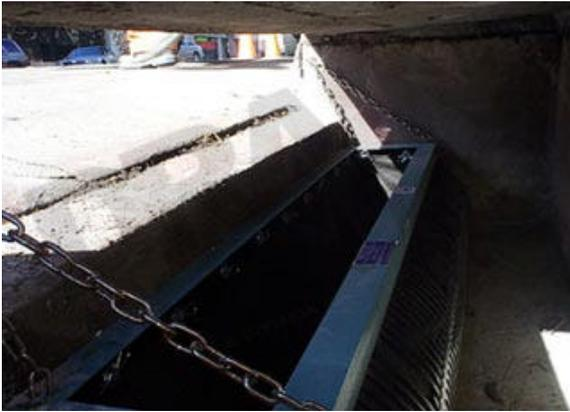
**Figure 3-13 DrainPac™ Insert**
