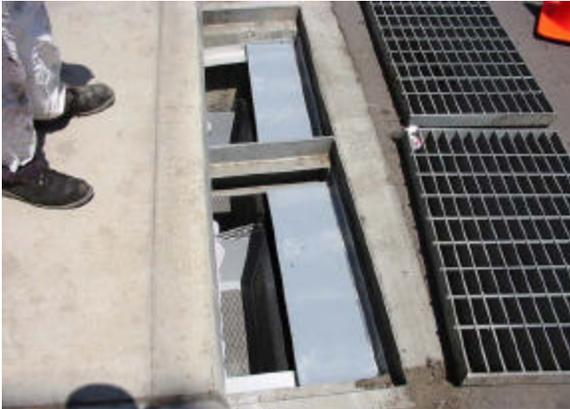
**Figure 3-15 BioClean™ Insert**
